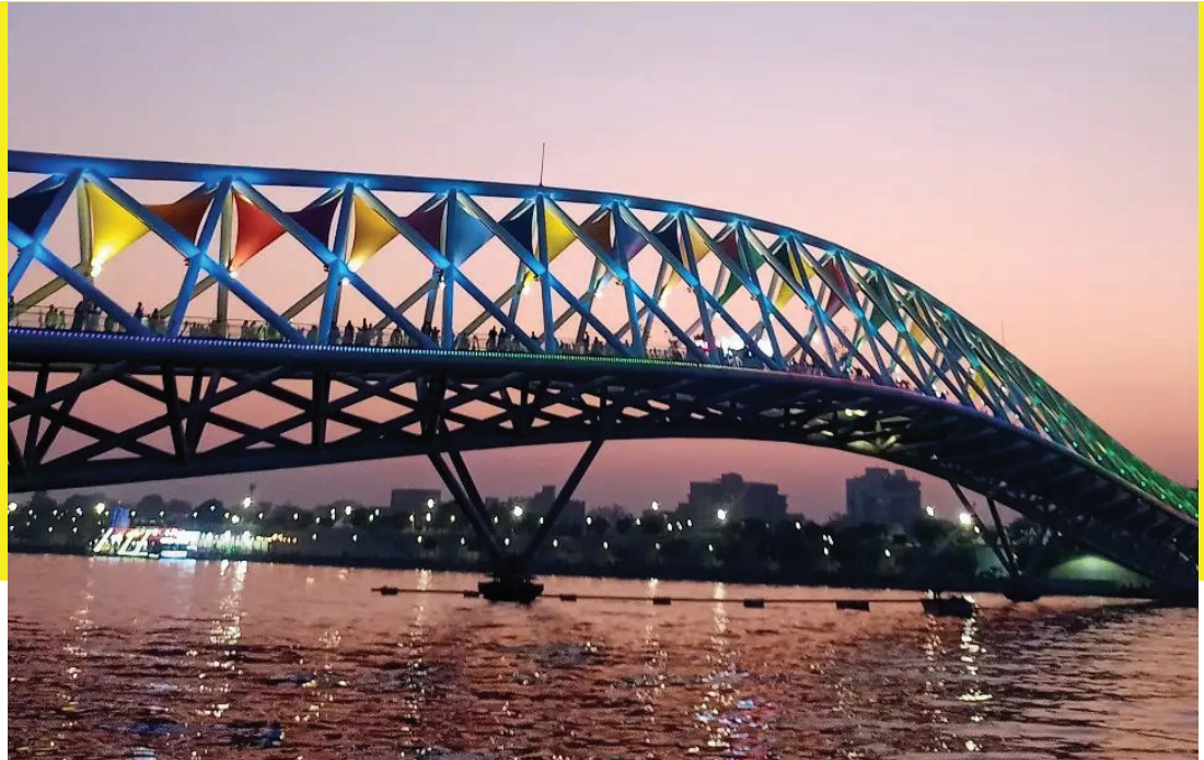
Atal Bridge, Ahmedabad
