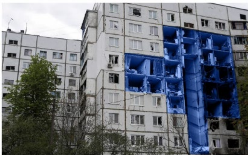
Figure 3. The SpeedStac in use in Ukraine (courtesy of WZMH Architects)
