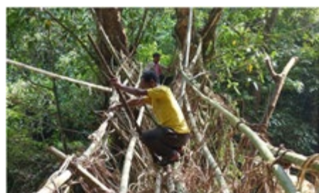
Figure 2. The living bridge construction from https://www.worldatlas.com/news/living-bridges-face-threats.html
