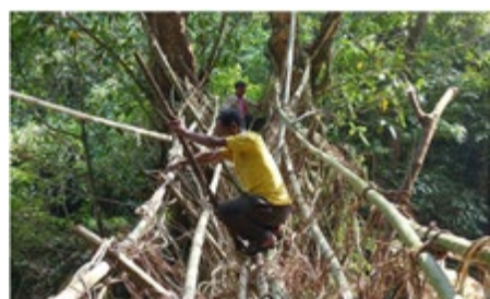
Figure 2. The living bridge construction from https://www.worldatlas.com/news/living-bridges-face-threats.html
