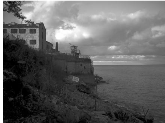
Figure 3. Battery prison, view from the city.
